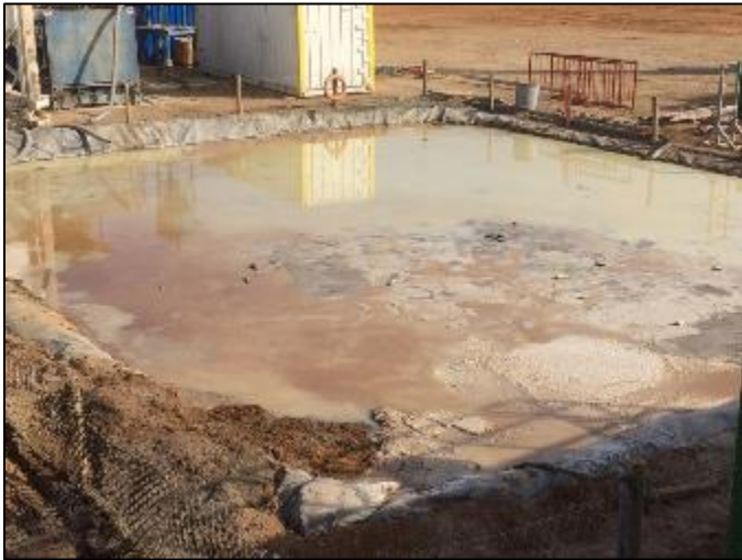
Fig. 02 – Remaining Waste Pit volume at Standard Dewatering System Rig Down (Well #2).
