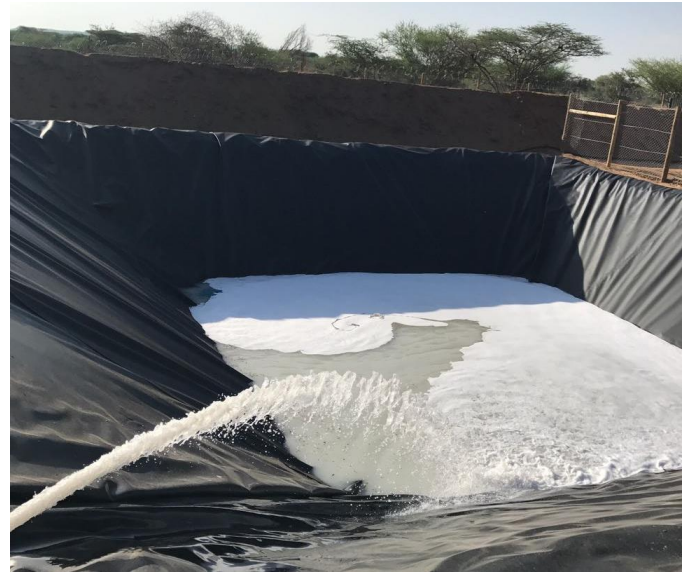
Fig 4 – Recovered Water from Dewatering. Pit capacity: 5,911 BBL. Note: The lack of water clarity is due to the addition of lime and biocide to reduce stagnation & degradation.
