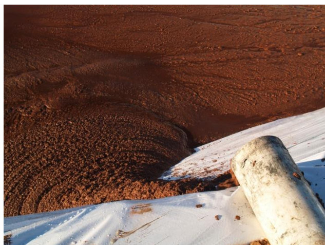
Figure 6: Dewatered Cuttings Output from DSSU
